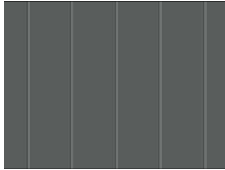
⑦ STANDING SEAM ROOFING, SOFFIT (OFFICE LEVEL)
