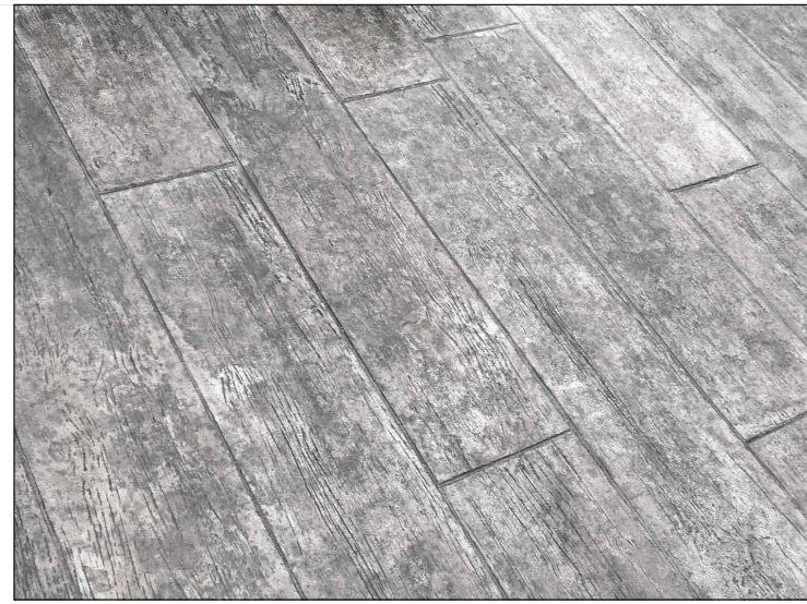
① STAMPED CONCRETE (PAVILION WALKWAY)
